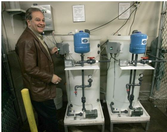
It turns out that zapping salt water with low-voltage electricity creates a couple of powerful yet nontoxic cleaning agents. Sodium ions are converted into sodium hydroxide, an alkaline liquid that cleans and degreases like detergent, but without the scrubbing bubbles. Chloride ions become hypochlorous acid, a potent disinfectant known as acid water.
